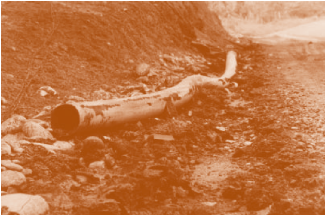
Oil pipeline, the target of bombing.
